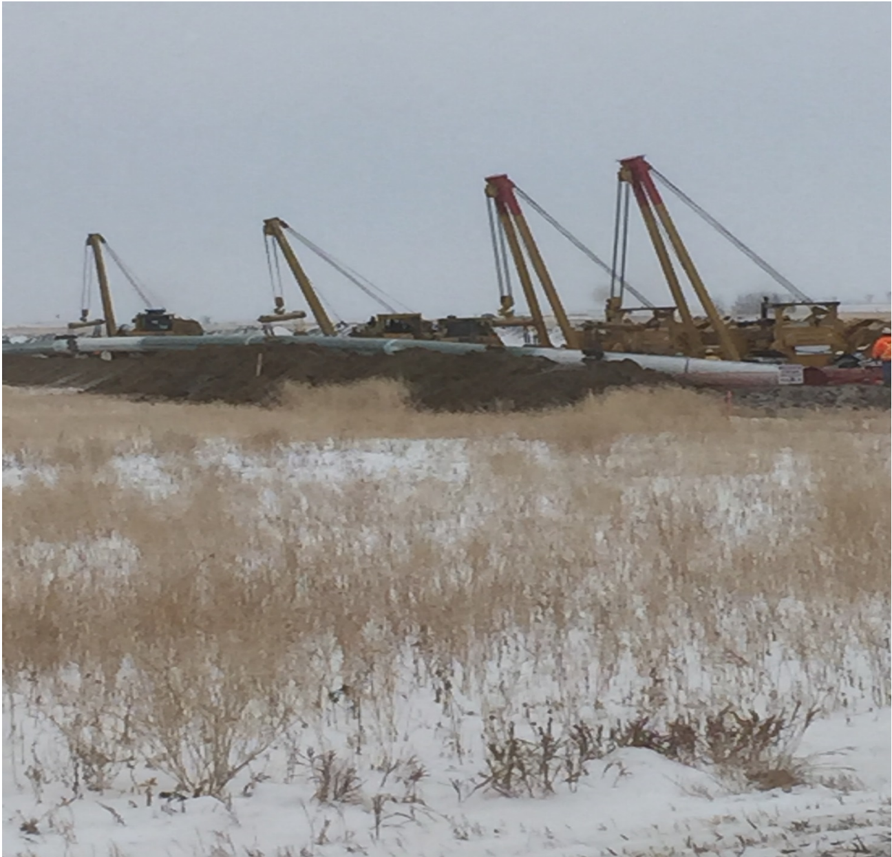
Lowering in crew
