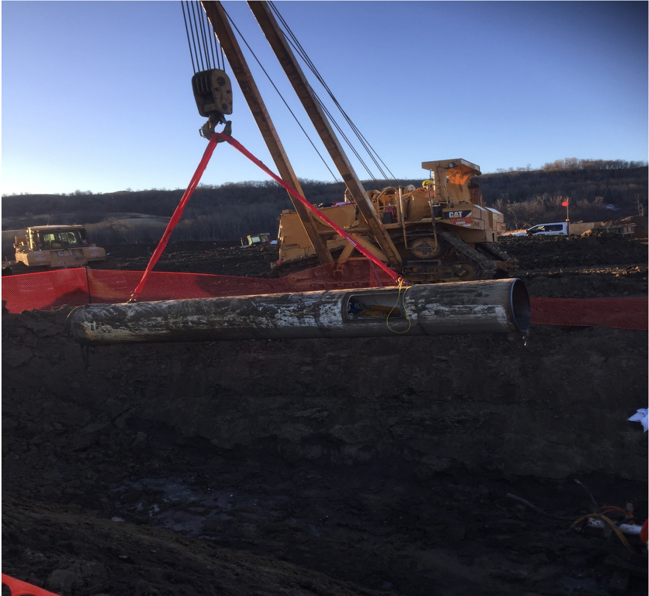
Specialised section of piping being lifted out.
